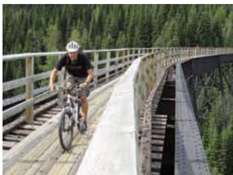
Photo: Bellevue Trestle, KVR – Martin Littlejohn
